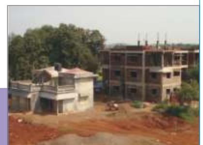
Principal & Staff Quarters (Under Construction)
