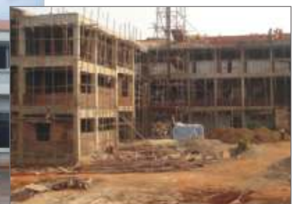
Institute Phase II under construction
